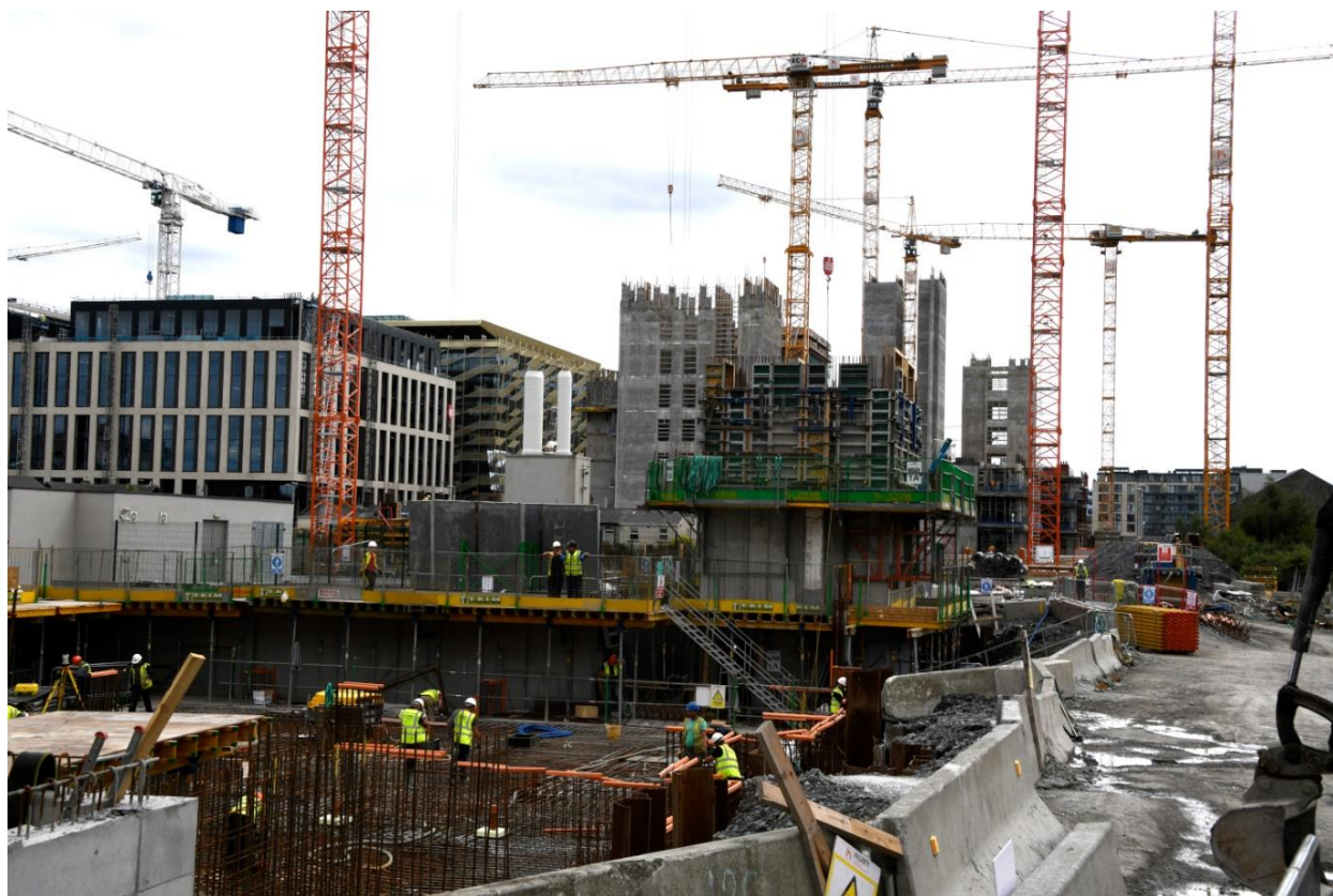
Plate 1. Ongoing Construction at the proposed development site (15 th August 2019).
